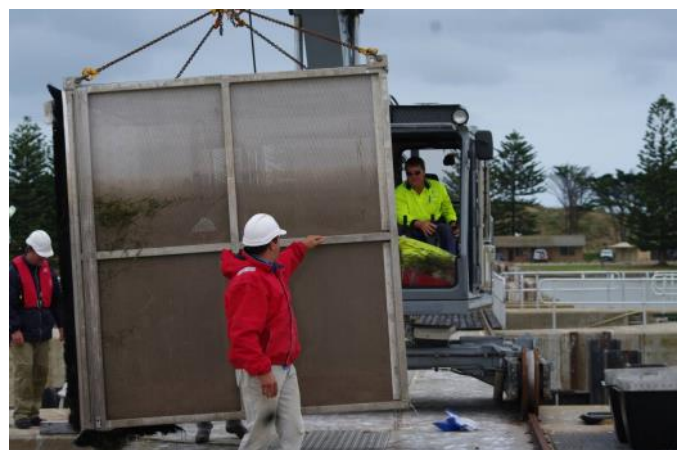
Installing the fishway cage trap at Goolwa Barrage (Adrienne Frears)
