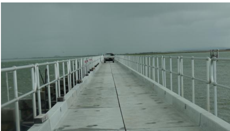
The Tauwitchere Barrage heading towards Ewe Island.
