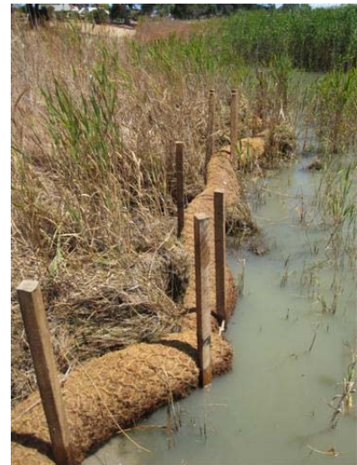
Coconut fibre logs preventing erosion
