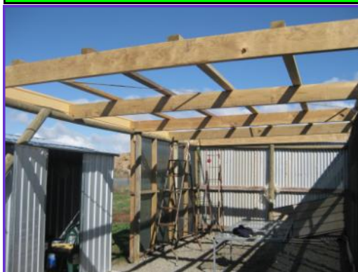
Undercover area under construction
